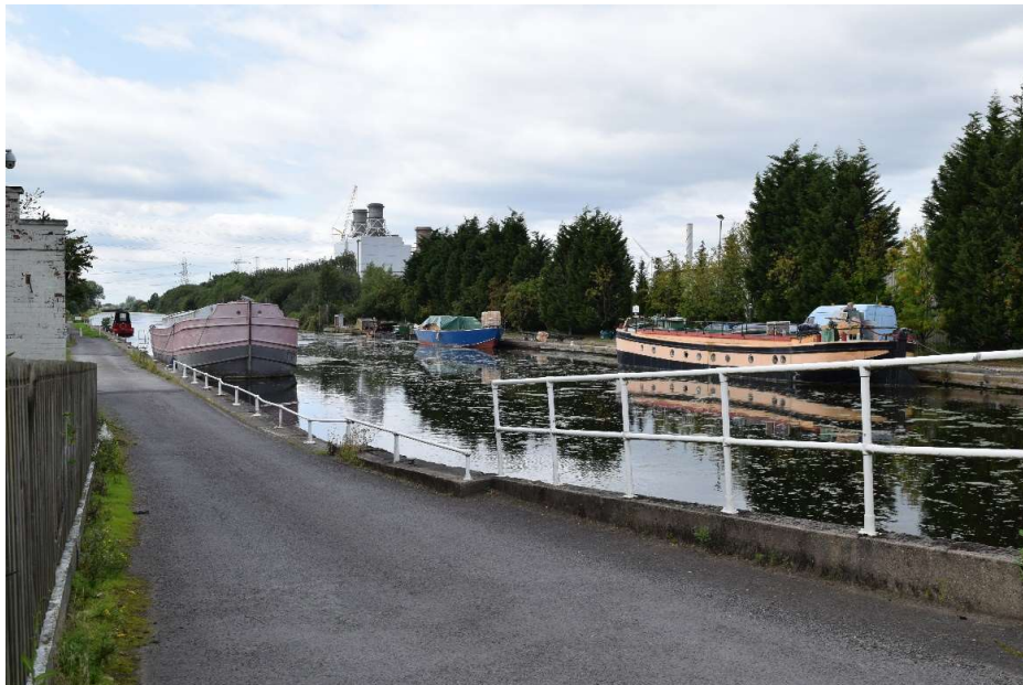
Plate 14: View along the canal to the west of Keadby Lock [NHLE1005204; NHLE1342734], featuring the existing Keadby 1 Power Station.
