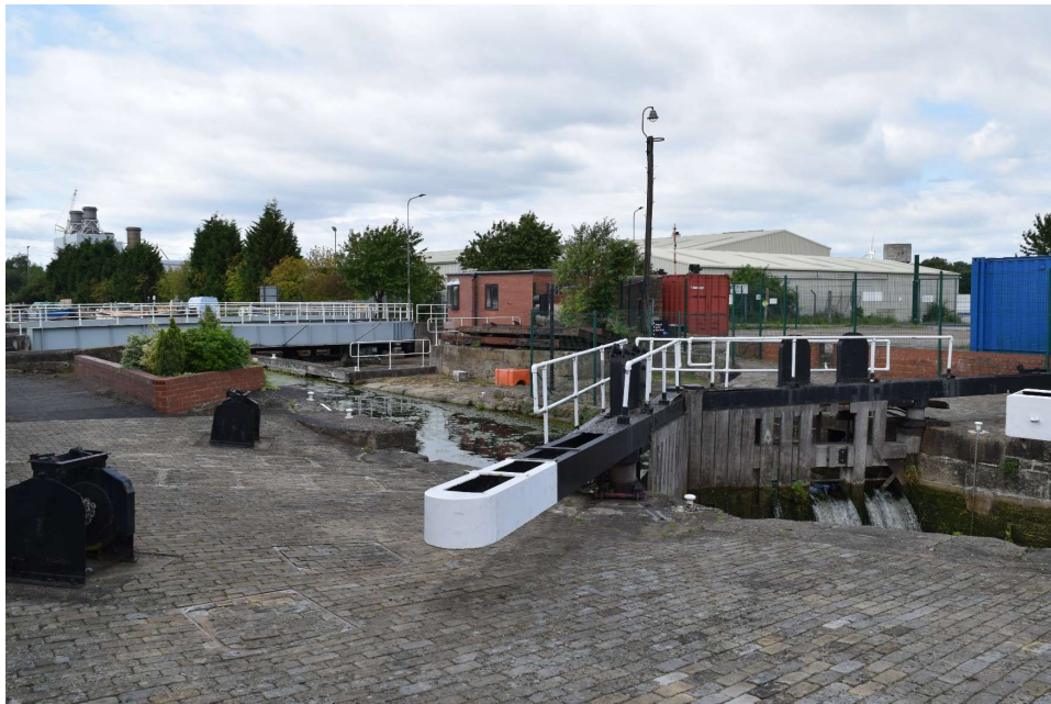
Plate 12: View north-west across Keadby Lock [NHLE1005204; NHLE1342734], with Keadby 1 Power Station visible in the background.
