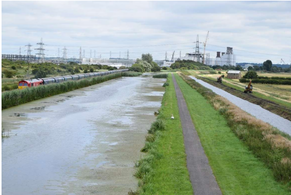
Plate 1: View of the North Soak Drain, Scunthorpe to Doncaster passenger rail line , Stainforth and Keadby Canal, and South Soak Drain (foreground), and Keadby 1 and 2 Power Stations (background) (north-east facing).
