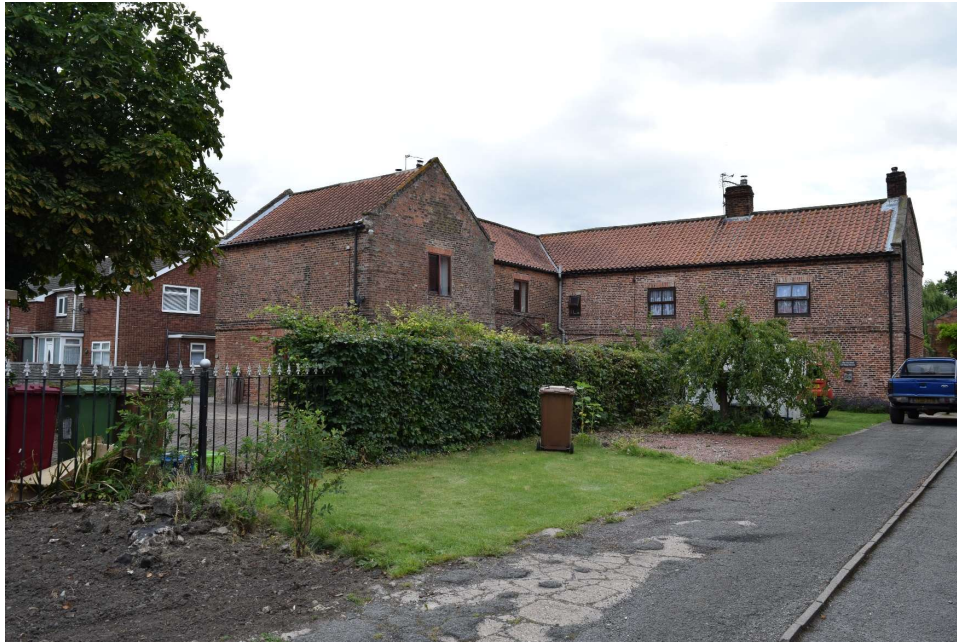
Plate 30: View of the Old Hall [NHLE1076980] in Althorpe, looking west.
