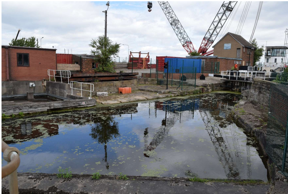
Plate 9: View east from the swing bridge overlooking Keadby Lock [NHLE1005204; NHLE1342734].
