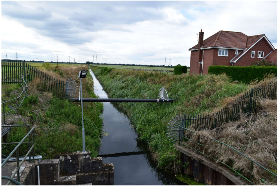
Plate 32: View along Warping Drain to the west of the Sluice in Derrythorpe.
