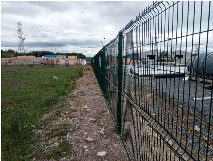
Plate 5: The existing laydown area, south of Keadby Common, on an area of prepared, made ground (north facing).
