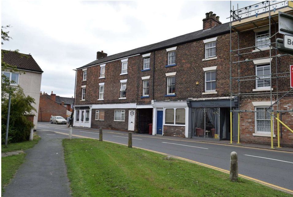
Plate 19: View south-west on High Street, showing the Grade II listed 2 Cross Street / 1-11 High Street [NHLE1083267].
