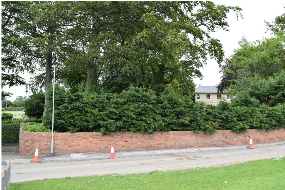
Plate 31: View of the Old Rectory [NHLE1083259] in Althorpe, looking west.
