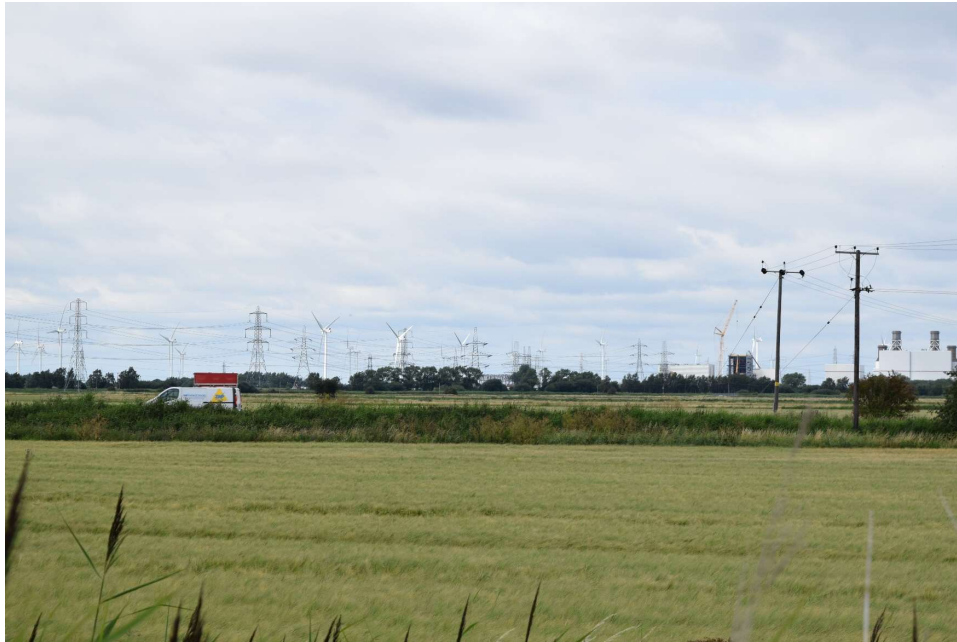
Plate 29: View from Crowle Bank Road featuring Keadby 1 Power Station, looking north.
